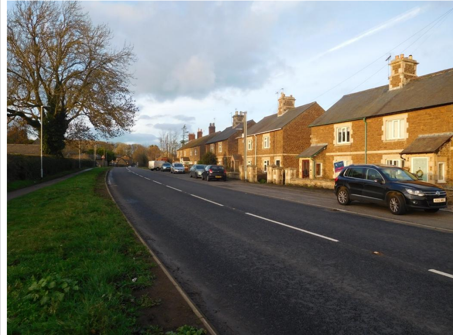
ID 2: The late-nineteenth century houses in Barleythorpe were built when the Earl of Lonsdale was the principal landowner.
