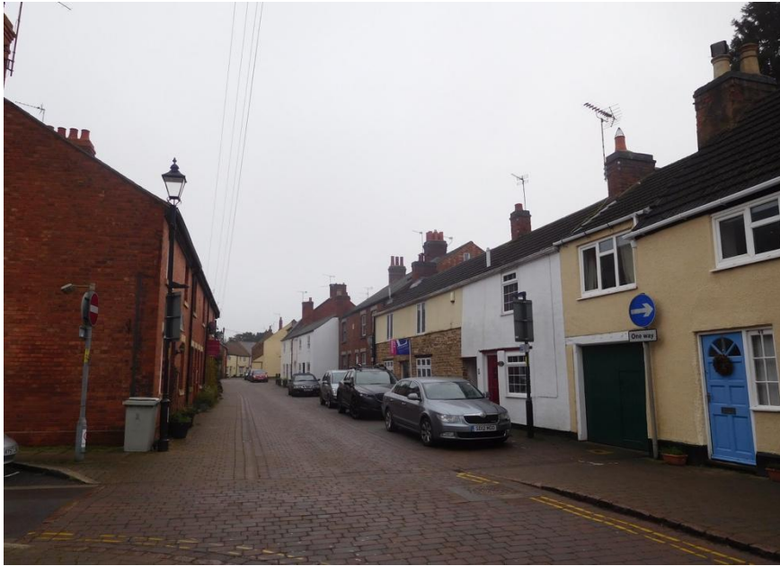
ID 7: Recent renovations enhance the attractive appearance has of Dean Street which mainly comprises late-nineteenth and early-twentieth-century terraces with older ironstone cottages which close off the further end.
