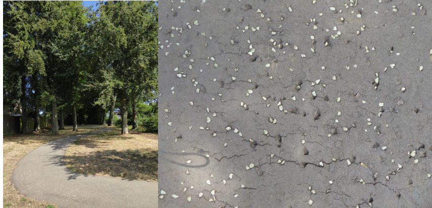
Footpath, including the fluorescent chips in the footpath, near Ashwell Road
