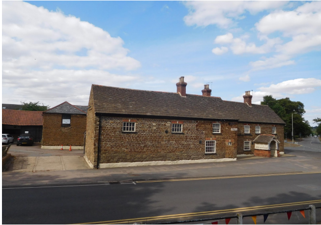
Station Road – Oakham School
