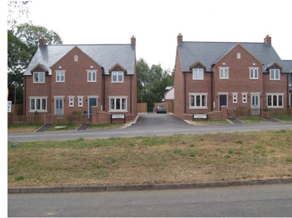
New infill housing on Braunston Road
