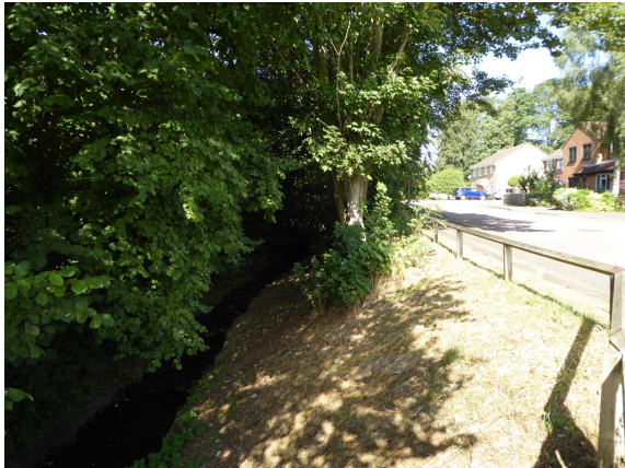
Barleythorpe Brook at Junction with Kestrel Road and Nightingale Way
